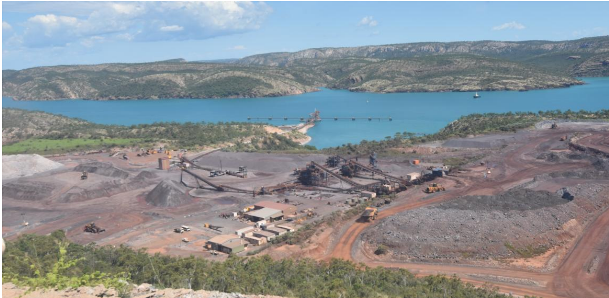
Figure 1 - Koolan Island processing plant and wharf (in background), March 2026
