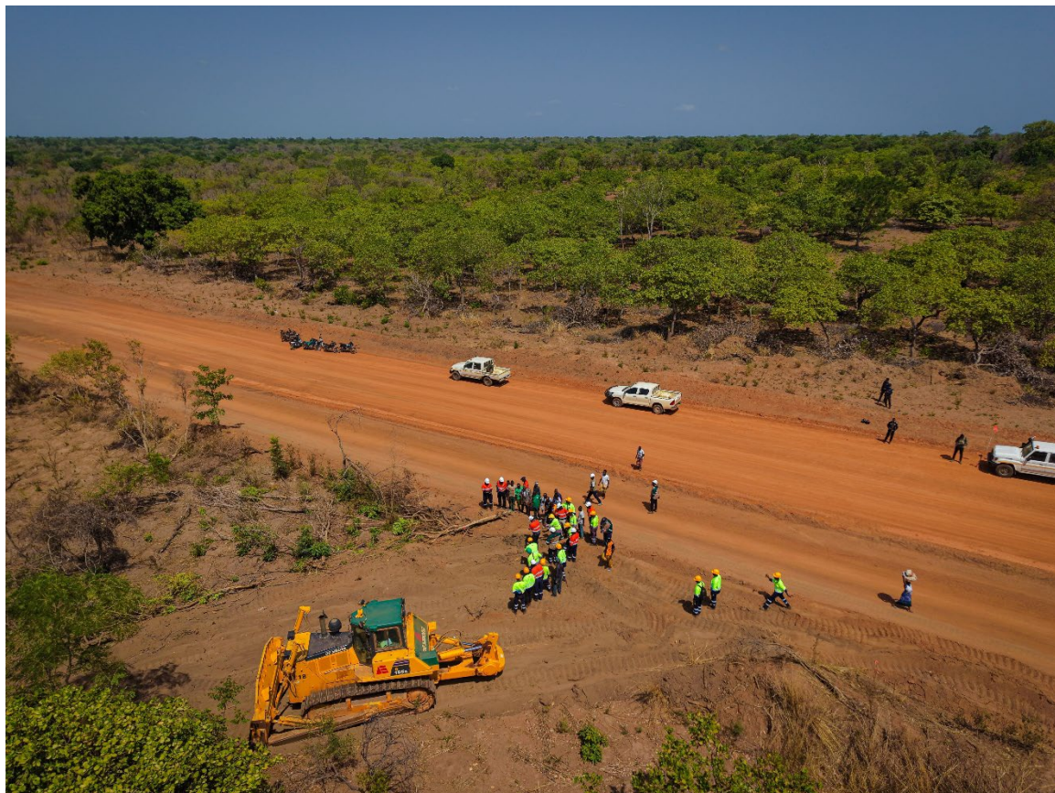
Figure 11: Ground clearance activities
