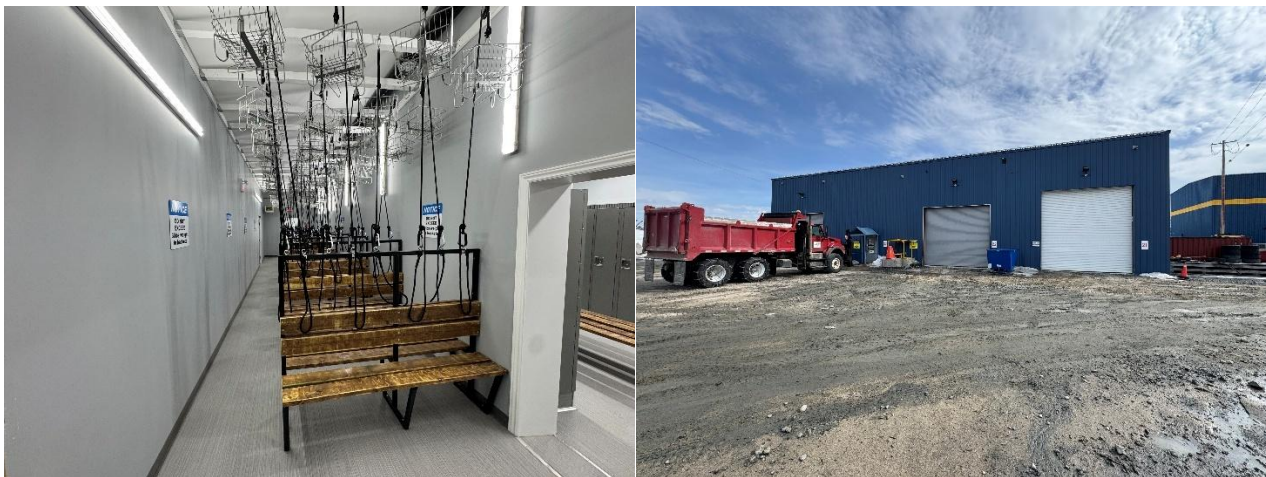
Figure 9: New changeroom facilities and maintenance workshop
