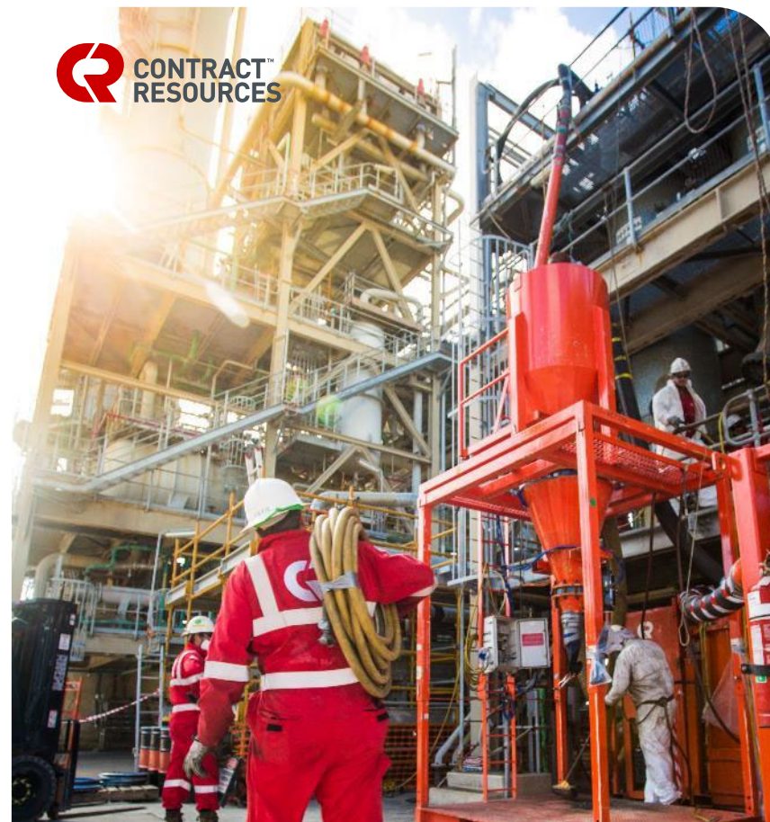
Pictured: Catalyst unloading at Ampol Lytton refinery supported by equipment setup on the ground
