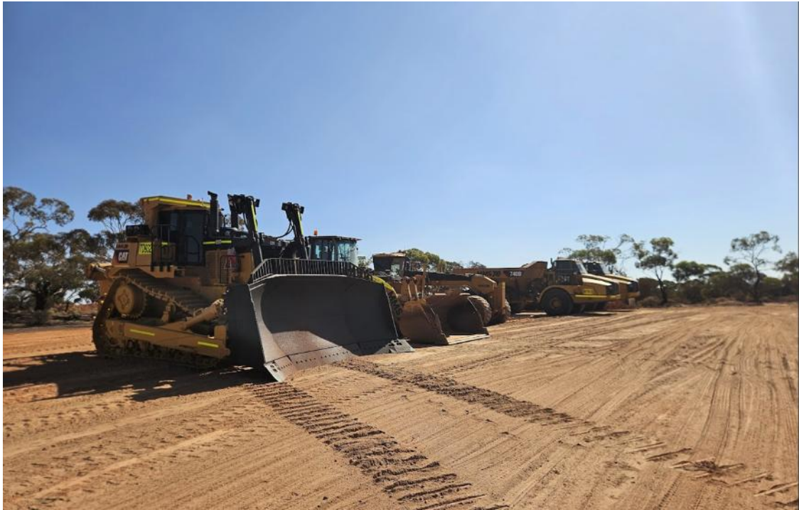
Figure 4– MMS mobilised at Waihi Open Pit operations
