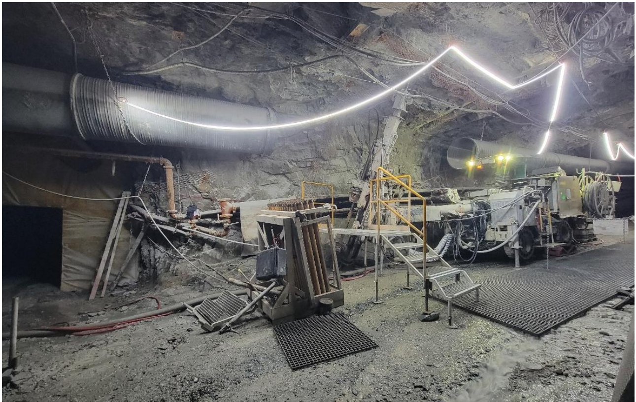
Figure 4: Drilling of DDH0289 against west rib, XC8.
