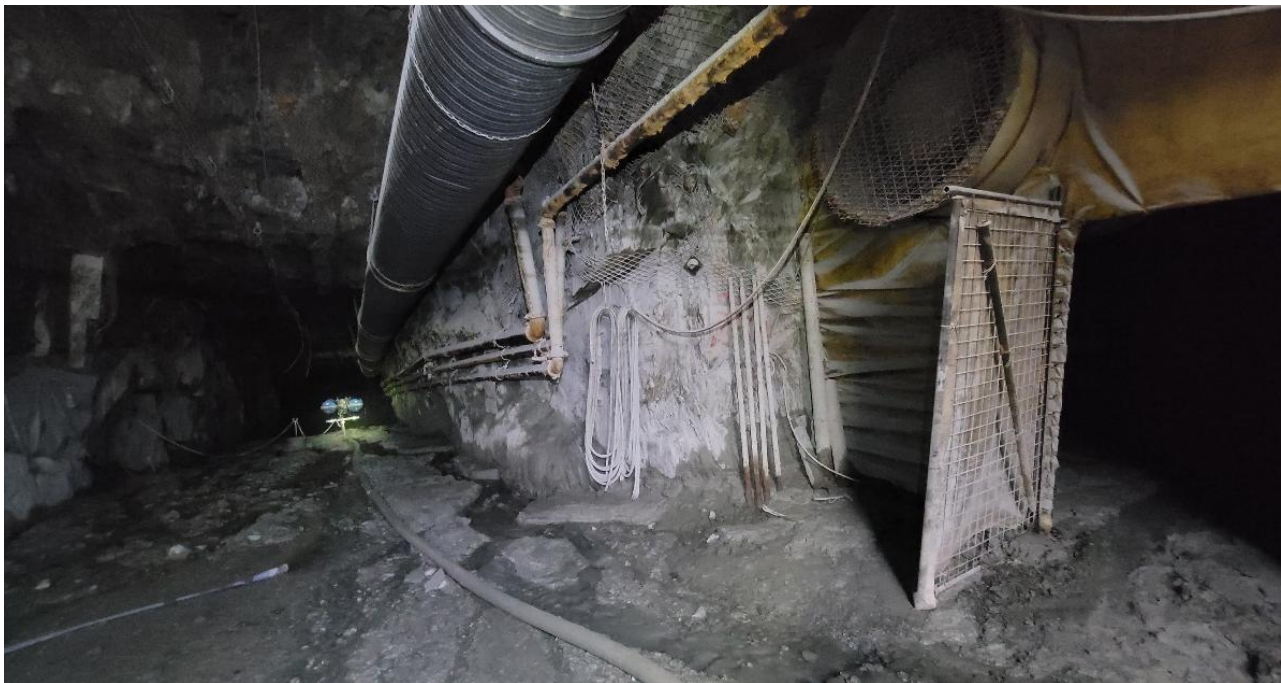
Figure 6: Dewatering continuing below XC8.
