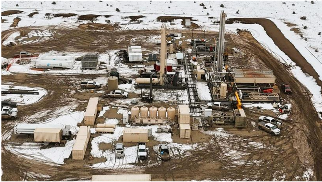
Figure 2: Construction of the Pinon Canyon processing plant
