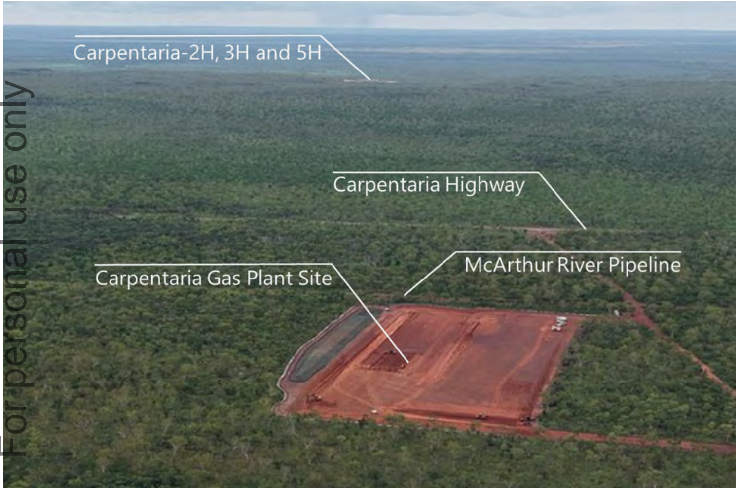
Civil works for the Carpentaria Gas Plant are complete
