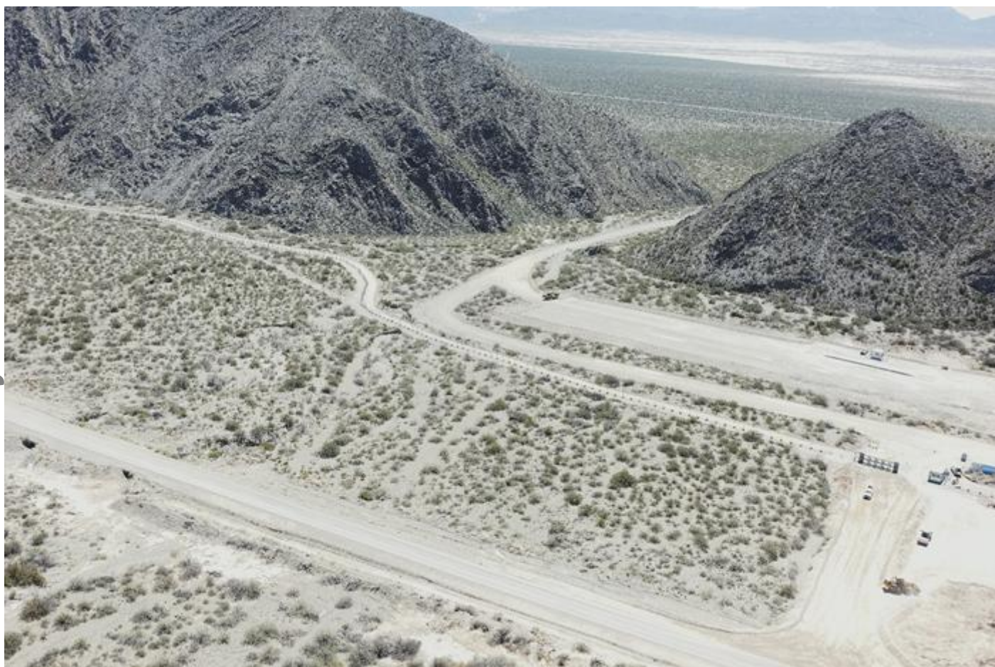
Figure 10- Main Access Gate as at 17 December 2025
