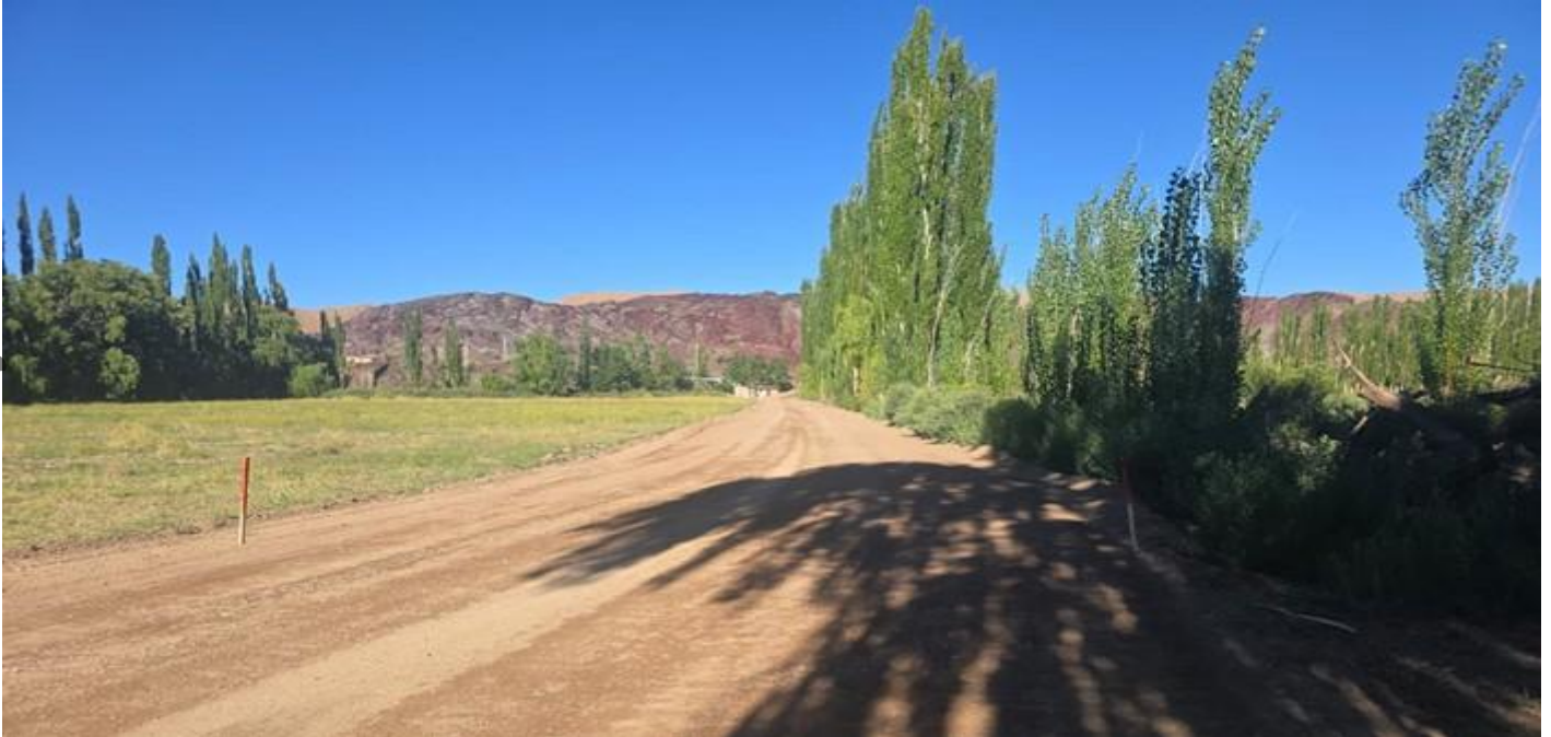
Figure 4 – Completed segment of Calingasta Bypass Road
