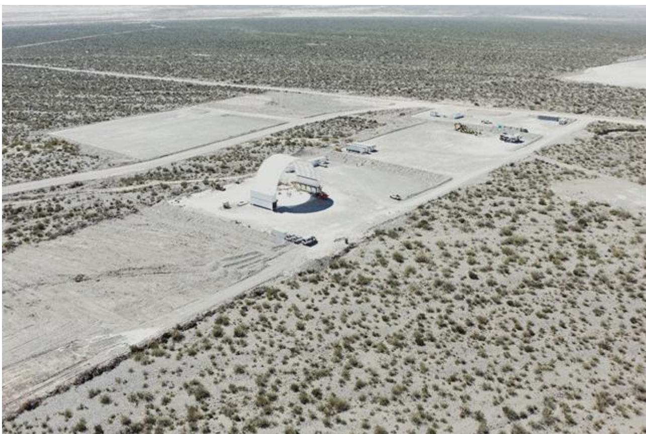
Figure 8 - Site Infrastructure Development as at 17 December 2025
