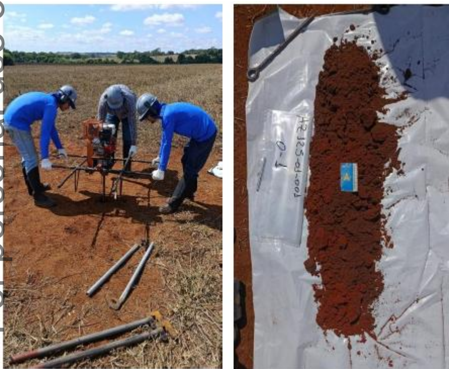
Figure 13 - Auger drilling is being undertaken by two three-man crews. Samples are collected at each 0.5m interval to a nominal depth of five metres at each site.
