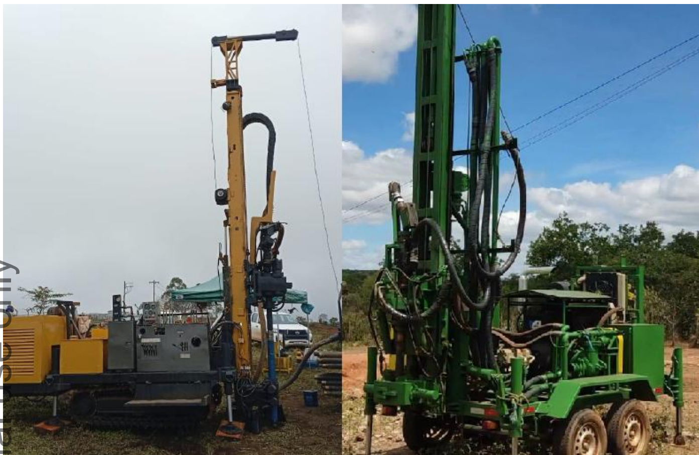
Figure 14 - 1st RC Drill rig to undertake drilling at Feirinha (left), 2nd RC Drill rig to undertake drilling at Feirinha (right).
