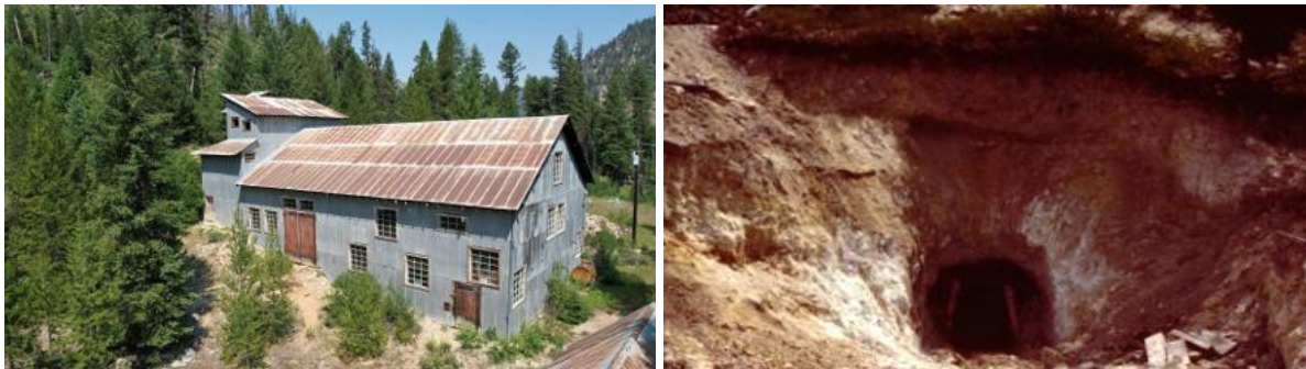
Figure 5: LEFT: Photo from the ASX Announcement of 2 March 2026 showing the Johnson Creek tungsten and antimony Mill. Refer also to Figure 3. RIGHT: Photo from the ASX Announcement of 2 March 2026 showing the adit of the closed tungsten mine at Golden Gate.
