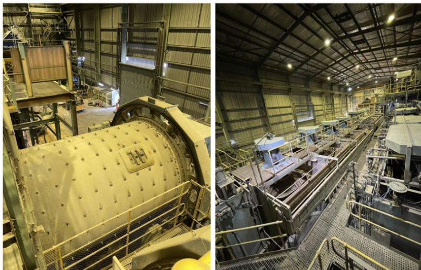
Figure 3. Ball mill and rougher/cleaner/scavenger units in mill.
