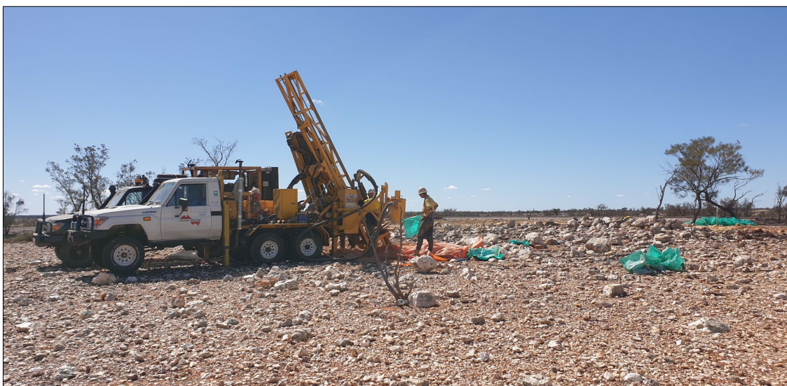
Photo 7. Aircore drill rig at the Bellagio Gold Prospect. Main quartz vein outcrop shown to the right of the drill rig. View towards north-east.
