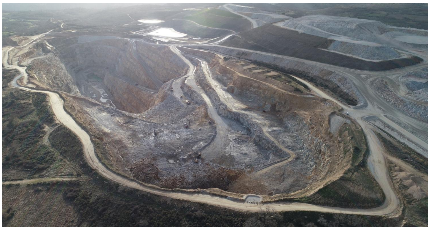
Barruecopardo Mine Open Pit, Northern Area. Phase 6 at elevation 680 RL, including the access ramp and 670 RL bench, with ore stockpile and waste dump on 31 December 2025.
