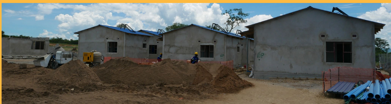
Work is progressing on the Tipume accommodation camp.
