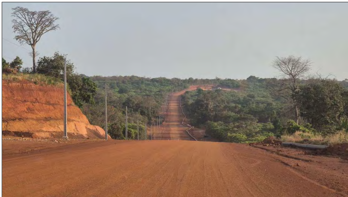
Figure 2.22: Mine to plant haul road
