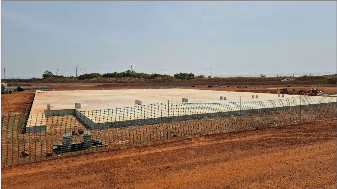
Figure 2.23: Koné mine hangar pad under construction
