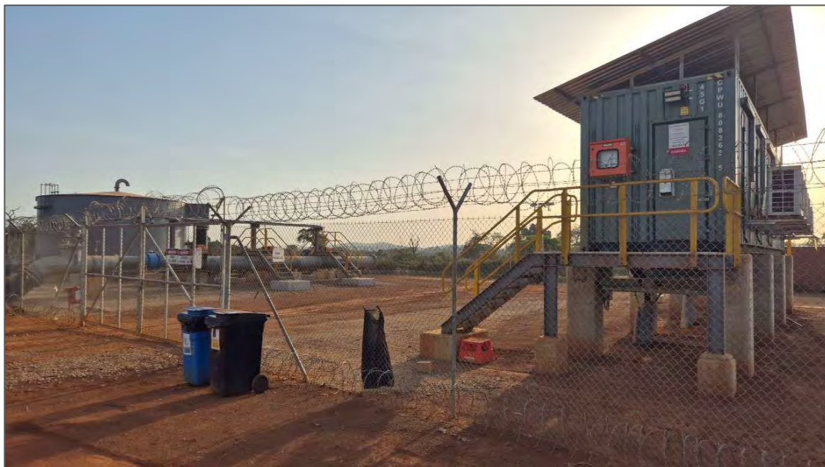
Figure 2.25: Water pump transfer station construction complete
