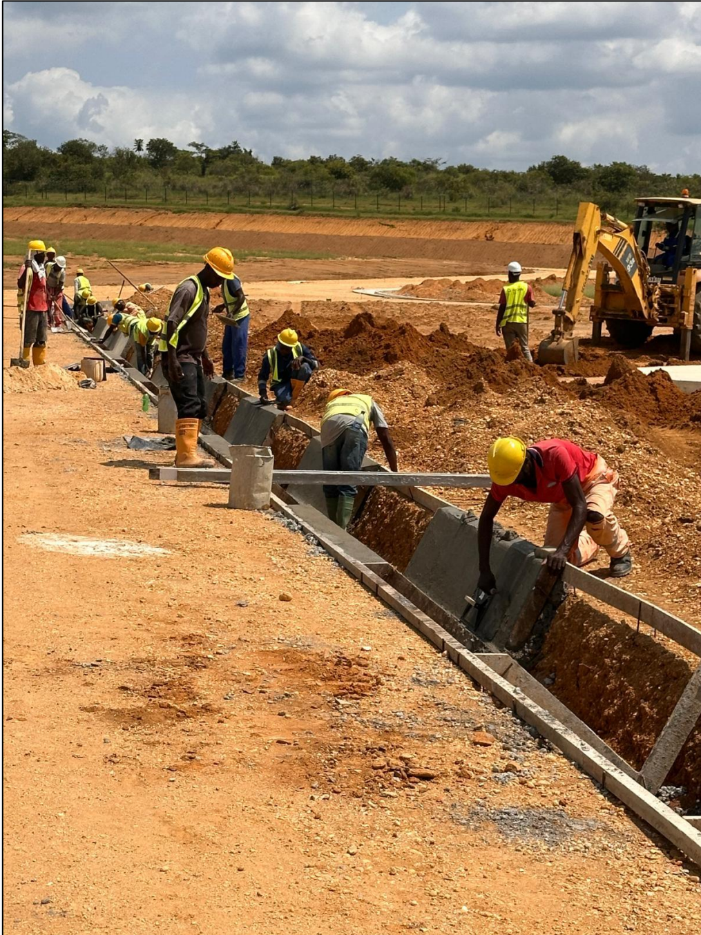
Figure 1 – Cabinda Phosphate Project, Angola with site works being completed during February 2026.
