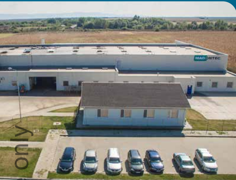
Magontec Romania Metal Recycling and Anodes Production facility
