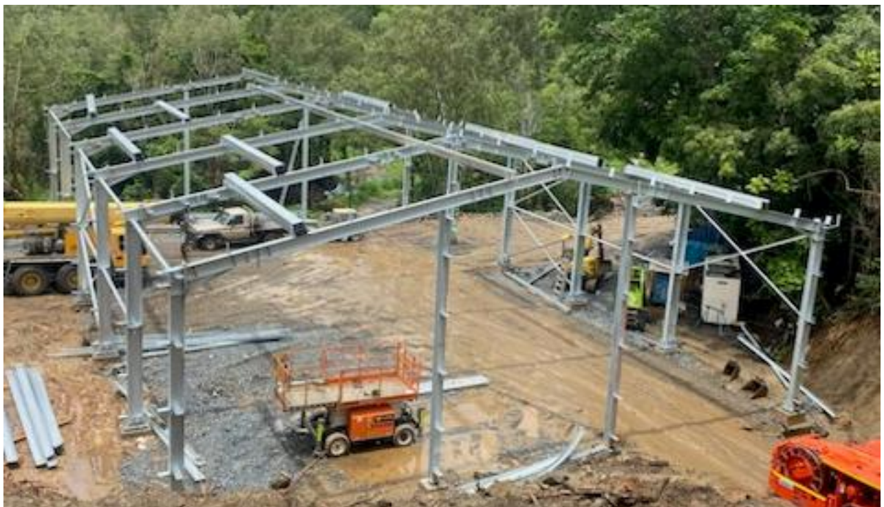
Figure 4. Acoustic load out facility construction.
