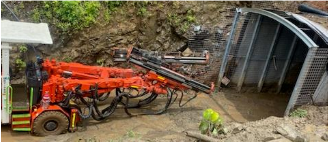
Figure 3. Development Jumbo Entering New Mine Portal at Dittmer
