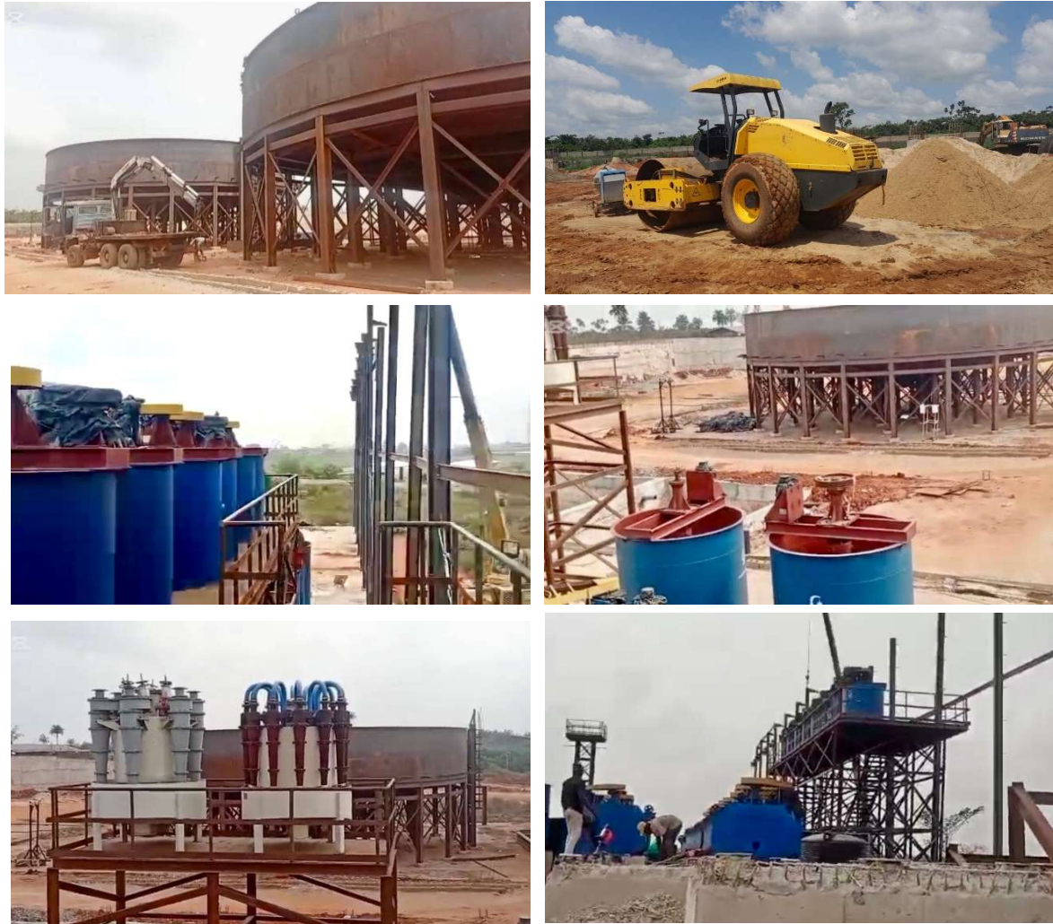
Photos of Construction of Norah Lithium Project Concentrator
