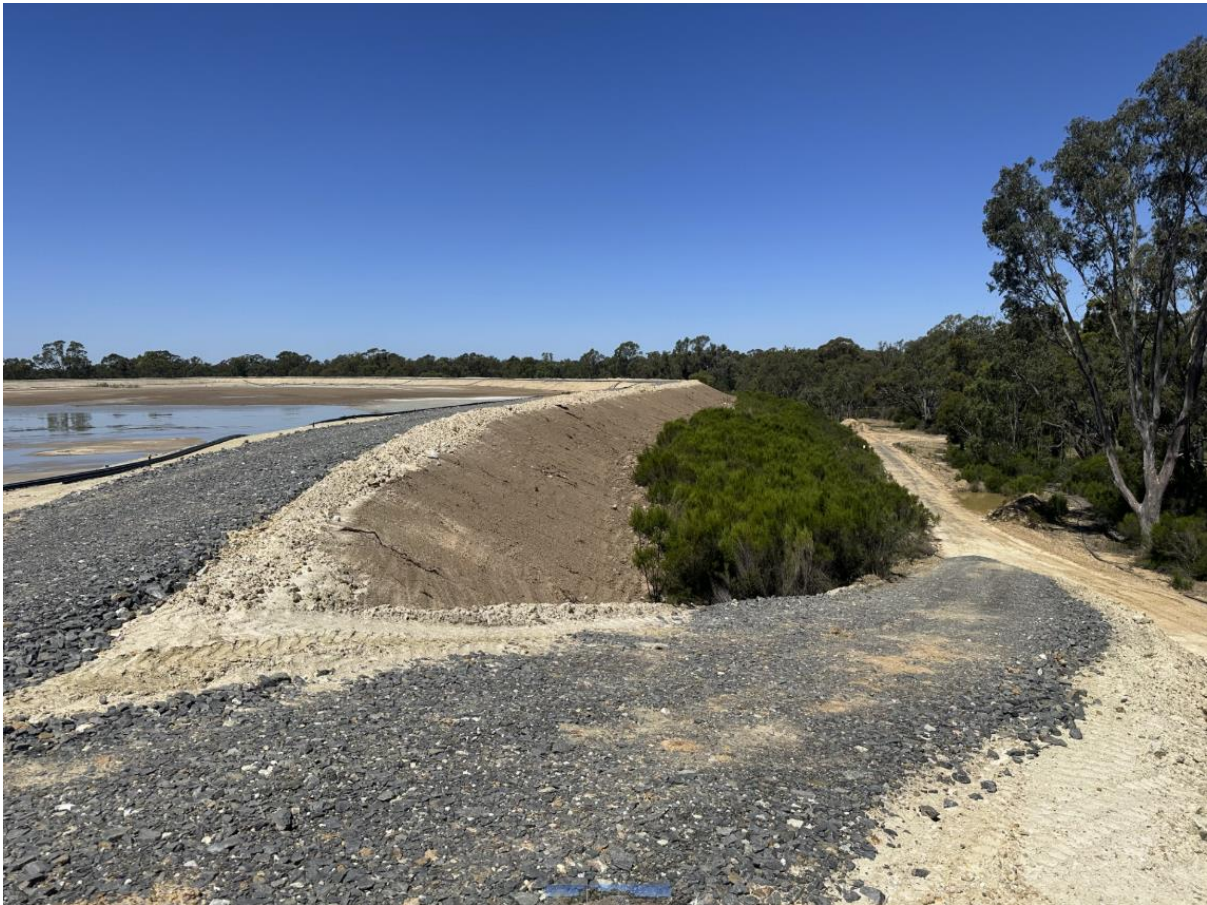
Figure 12. Tailings Storage Facility lift 5 D completion
