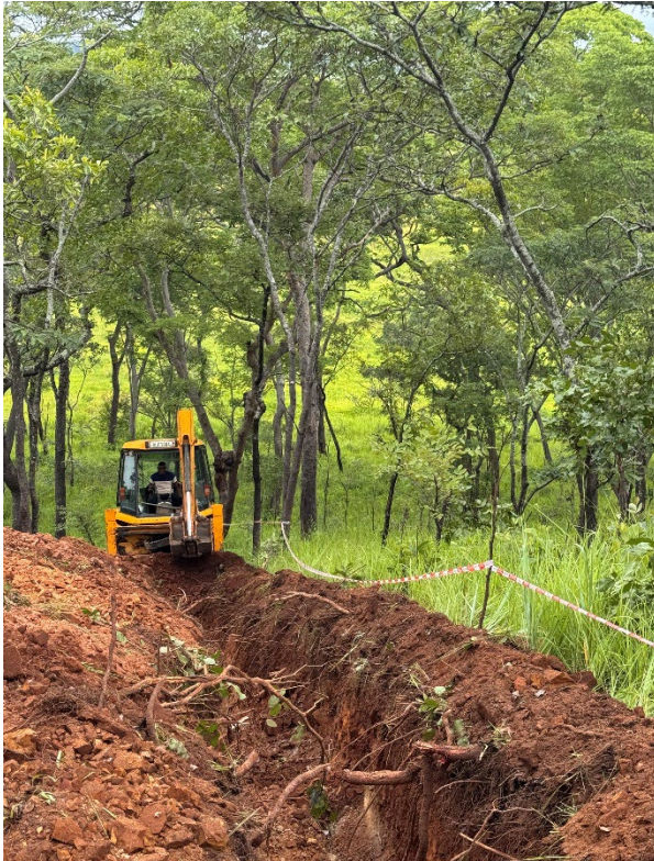
Figure 2: JCB Backhaul loader excavating trench TBTR05
