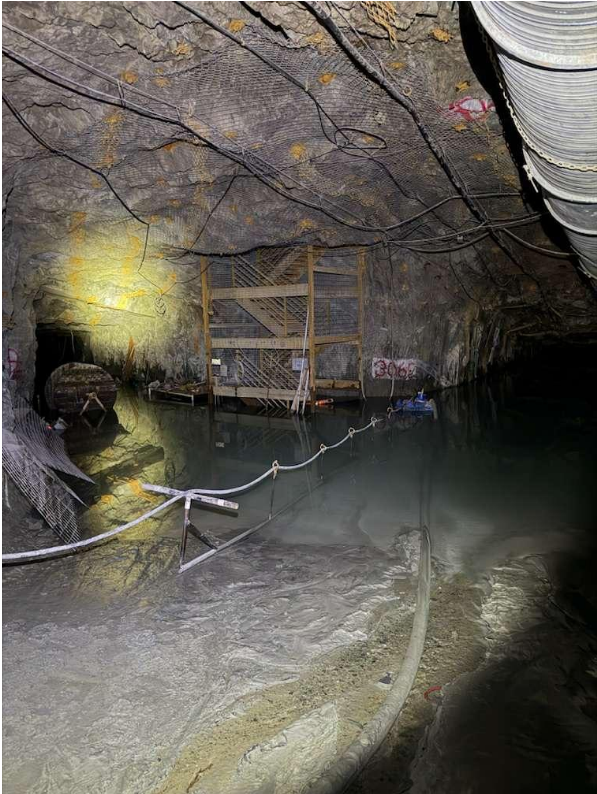
Figure 3: Dewatering progress at Stringbean Alley Decline. XC5 viewed looking east. Pump (blue) is currently draining the remaining water from the crosscut. Stairs up to 1030 development drive in mid-shot. Picture taken 18 January 2026 Pacific Standard Time (PST).
