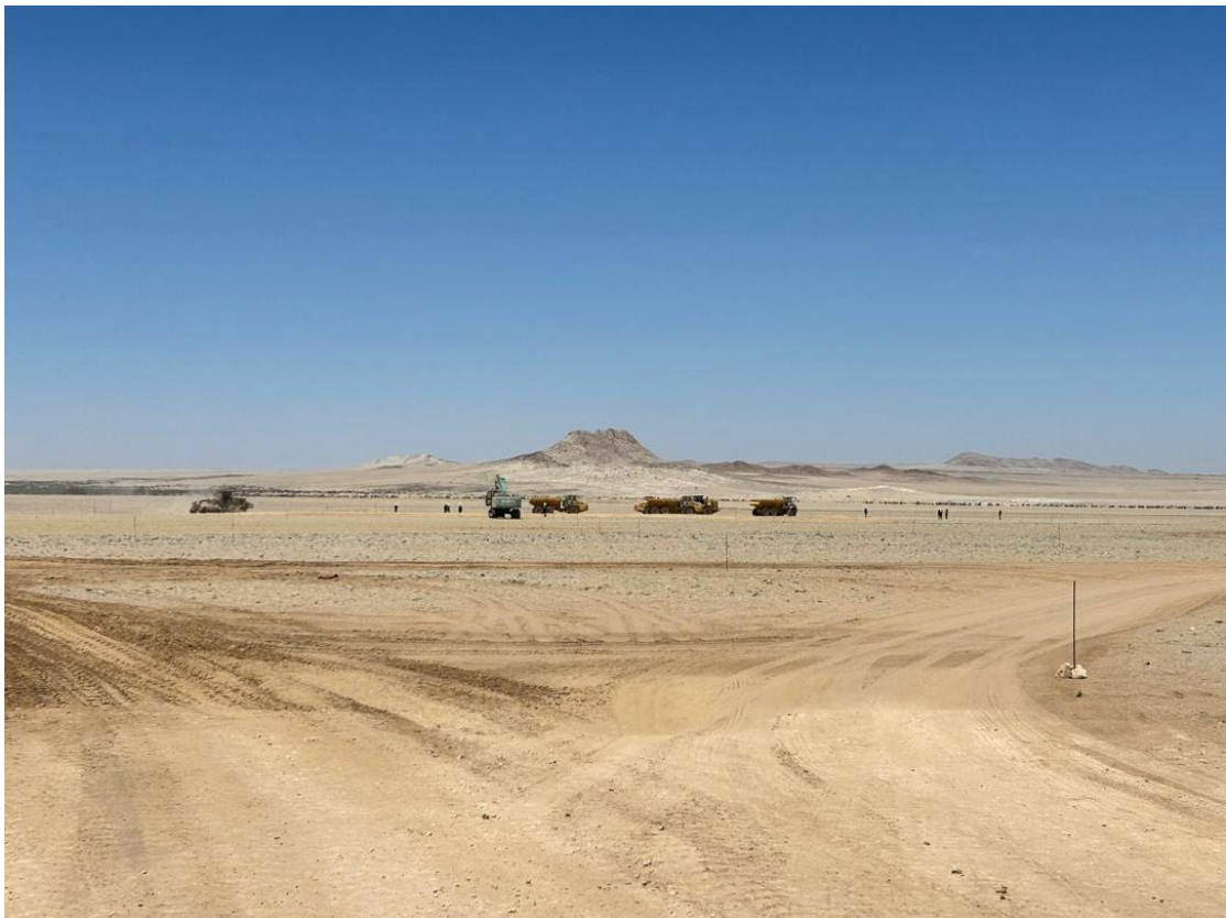
Figure 3: Bulk earthworks contractor stripping topsoil.
