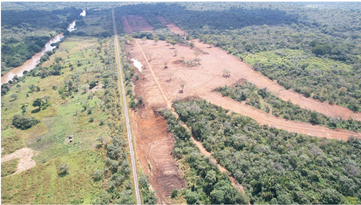
Image 4: Inland Rail Facility Earthworks
