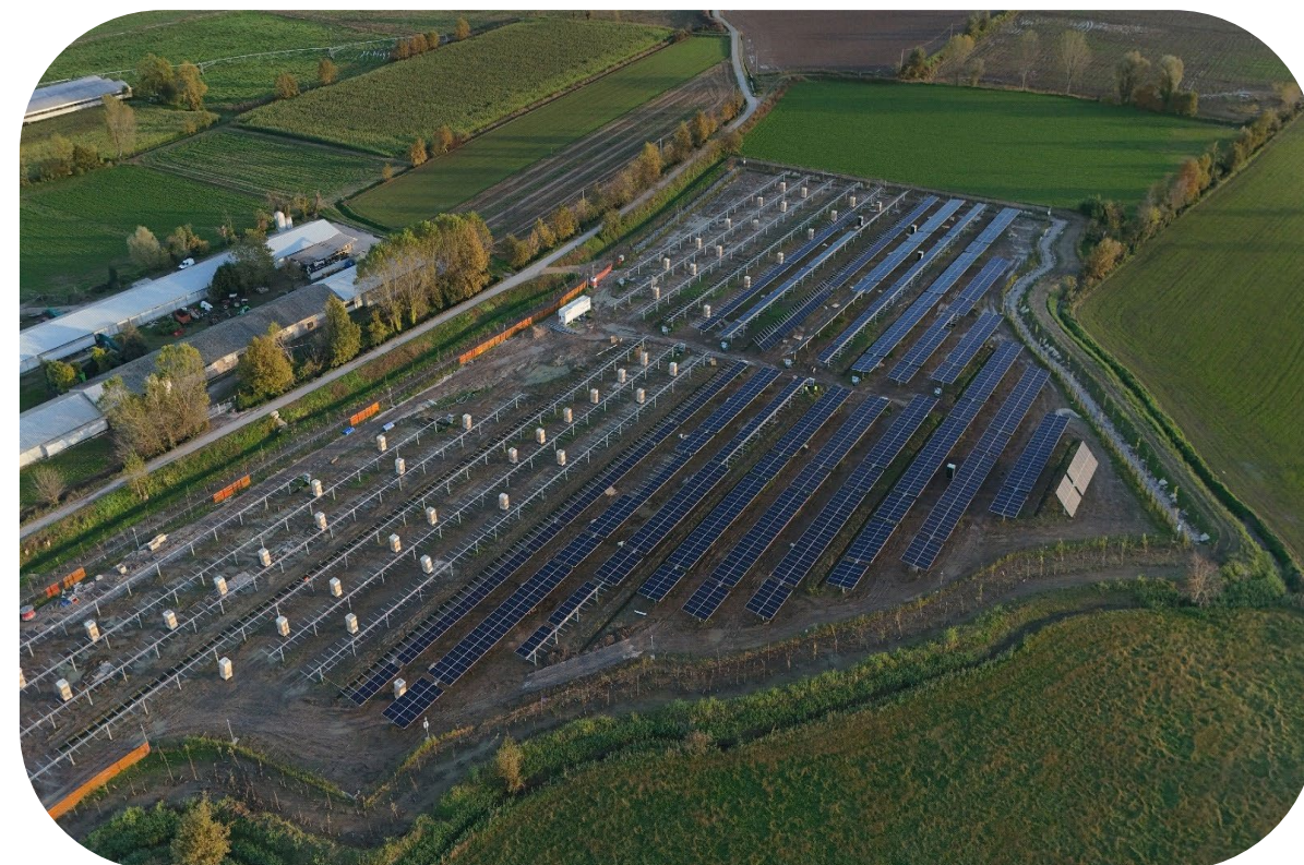
Galileo's solar project under construction in the Lombardy region, Italy.
