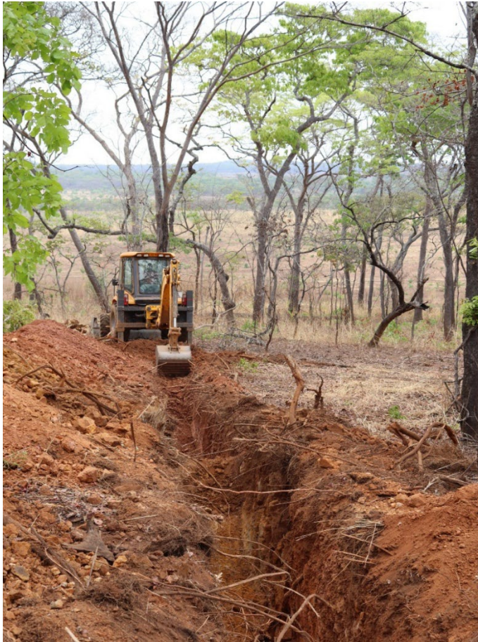
Figure 2: Mahindra SX90 TLB trenching on TBTR03.
