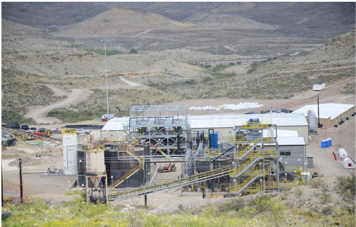
Figure 5: Shafter Processing Infrastructure.
