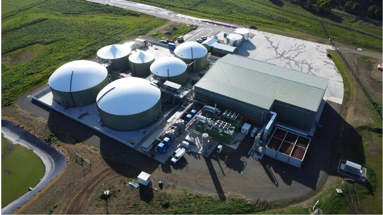
Yarra Valley Water Bioenergy plant in Lilydale
