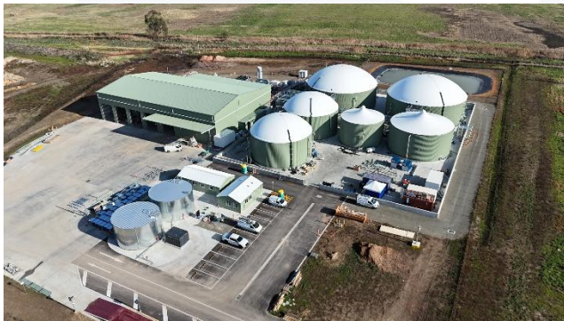
Yarra Valley Water Bioenergy plant in Lilydale
