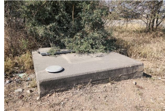
Water Source at Entrance
