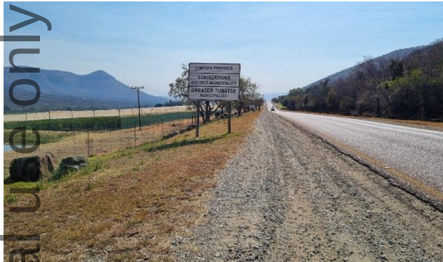
Paved Road to Site
