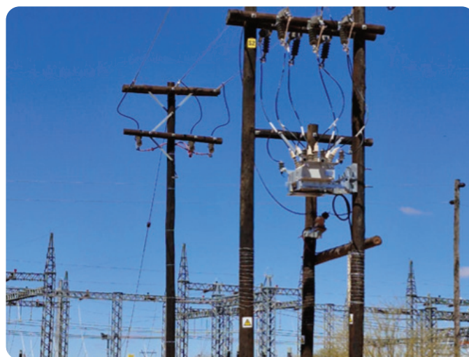
Photo 5: Cuprum Substation 15MVA tie-in to PCZM electrical reticulation.
