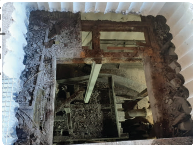
Photo 4: Hutchings Shaft Cement Slab Opened.
