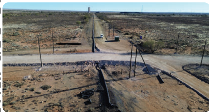
Photo 3: Dewatering Pipe and Overhead 11kV to TSF.
