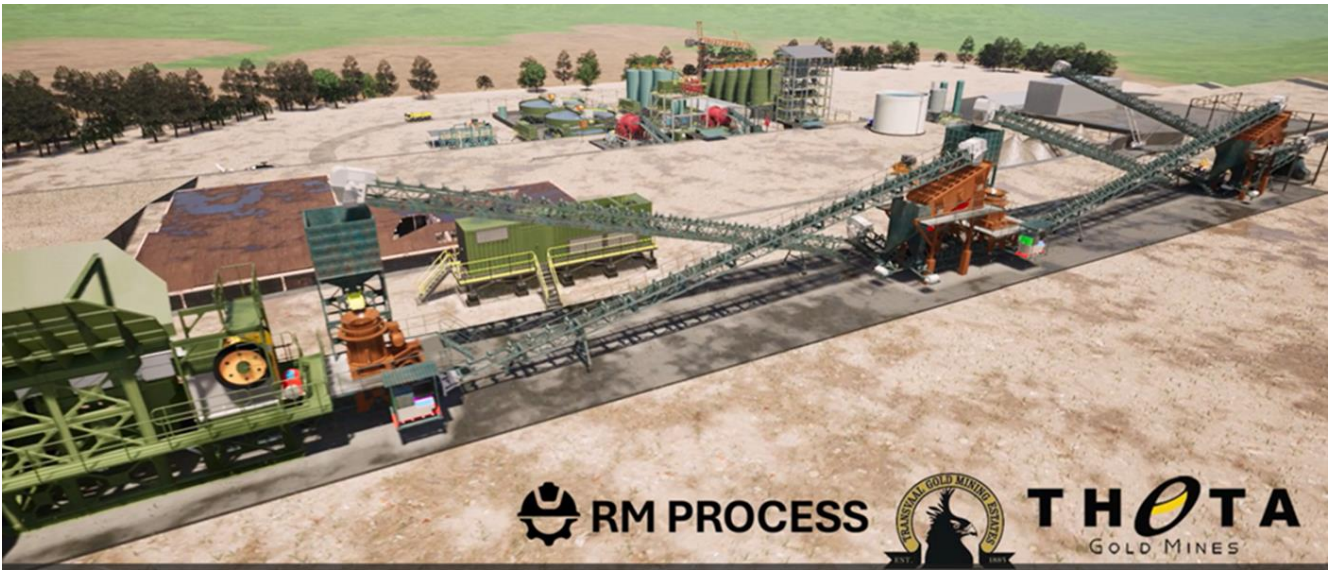
Figure 19: 3D rendering by RM Process of the Crushing Circuit in Foreground
