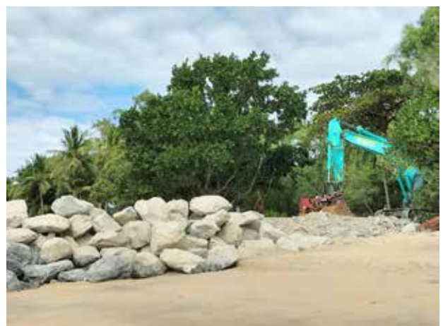
Mt Carbine Quarry armor rock used on the Cairns Northern Beaches for boat ramps, beach protection and jetty.
