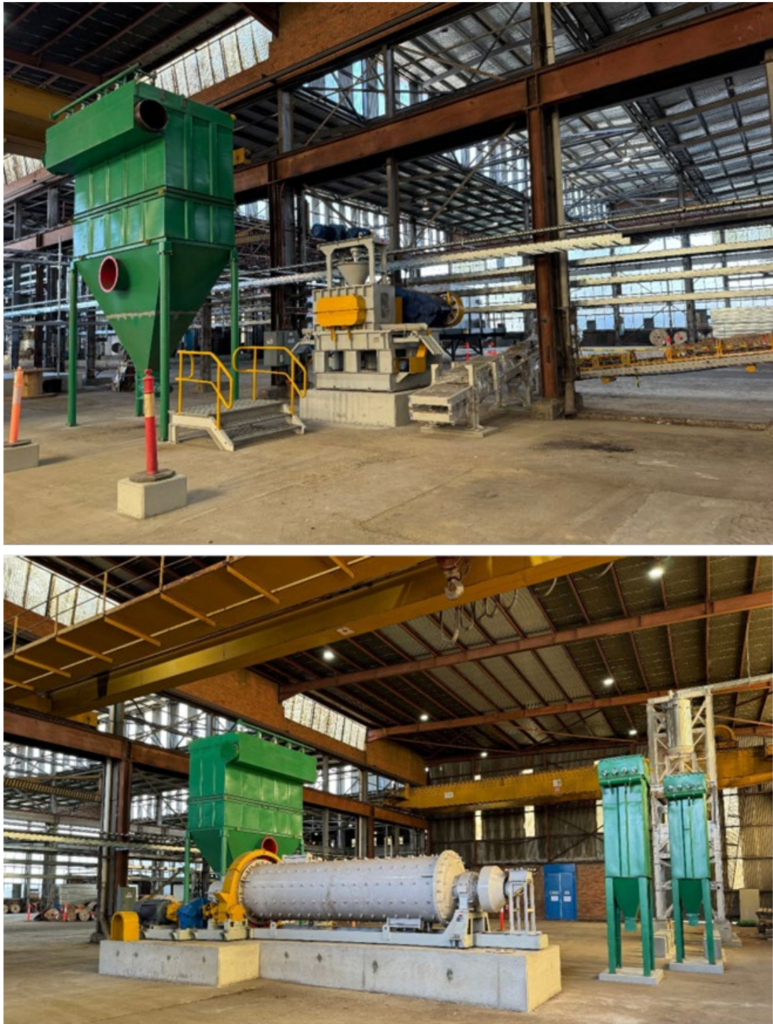
Figure: Briquette civil work completed with major equipment set in position on foundations
