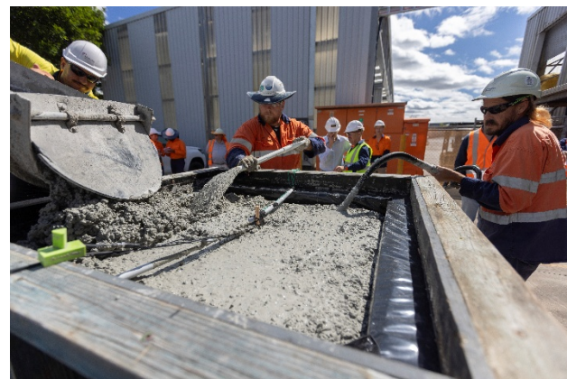
Figure 5: AusPozz™ concrete hotbox demonstration pour and temperature monitoring
