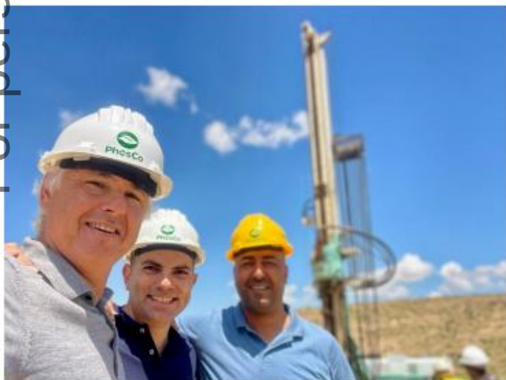
Photo 2: Drilling underway at GS Prospect
