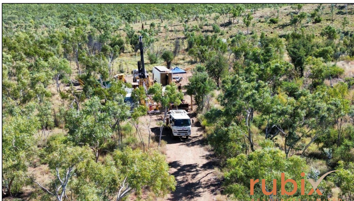
Figure 3 – Aerial view of the drill site at Grunter north, showing the compact footprint of the site.
