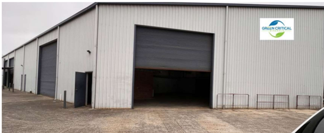
Figure 1 - GCM VHD Technology Industrial Facility
