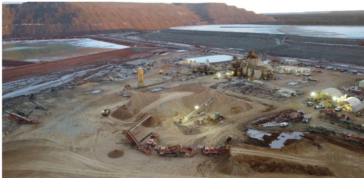
Figure 11: Lakewood Processing facility
