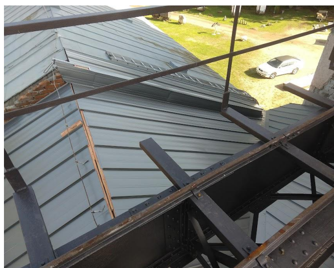
Image 3 (left): cleaning and painting the rail link bridge over the engine room; Image 4 (right): near complete roof repairs and installation on the engine room at the Sturec project;
