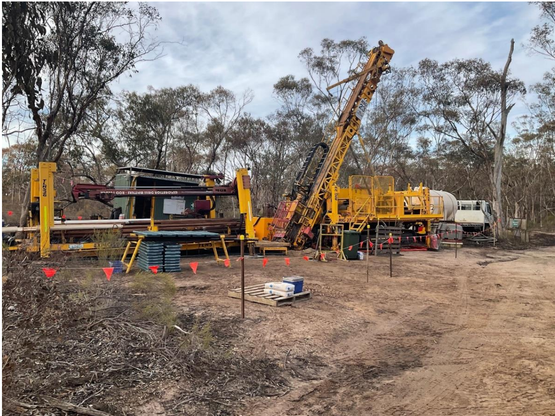
Figure 2: Drilling at Crosbie South.
