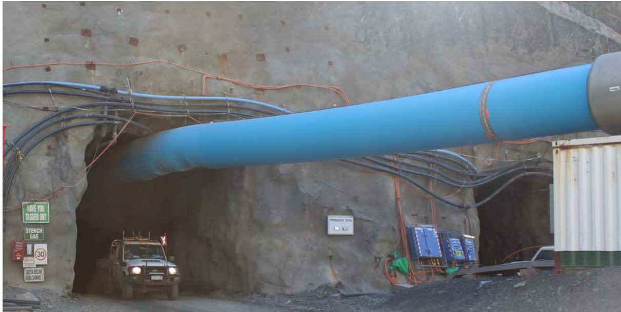
Picture – Scotia Underground Mine, South Portal.
