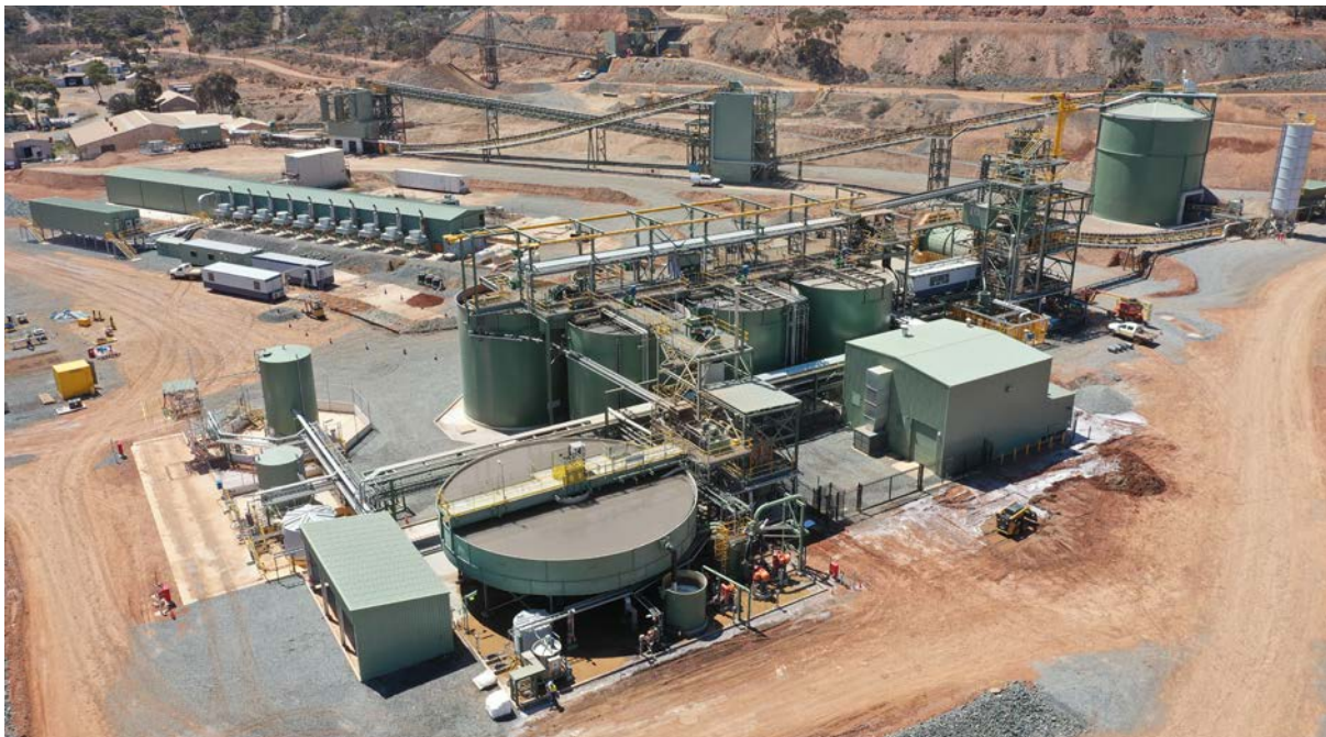
Picture – Norseman Processing Facility.
