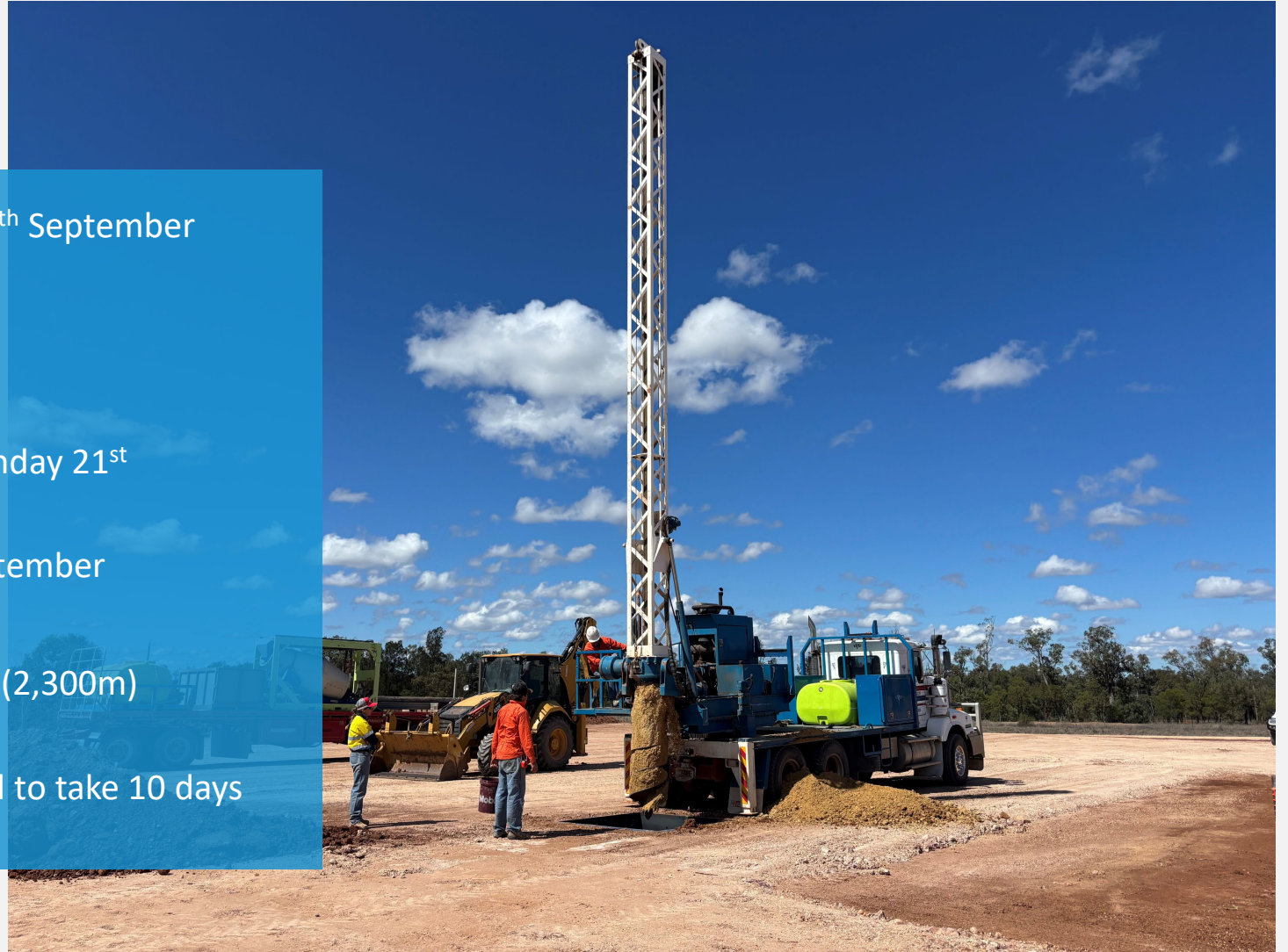
Installation of the Conductor pipe at Diona-1
