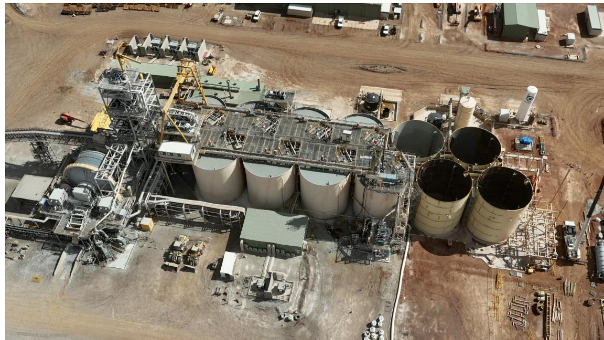
Absorption tanks
