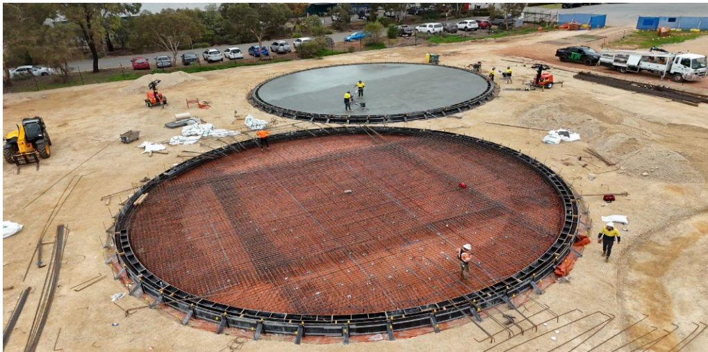
SA1 Salisbury Bioenergy construction
