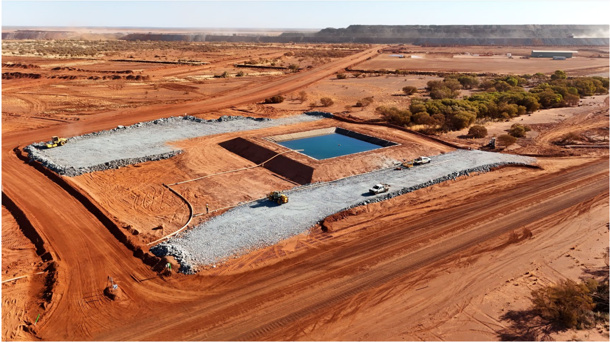
KEP Berwick Pit Dewatering Turkeys Nest
