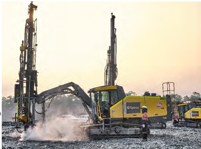
Figure 5 | Epiroc T-45 Blast Hole Drills at Okvau
