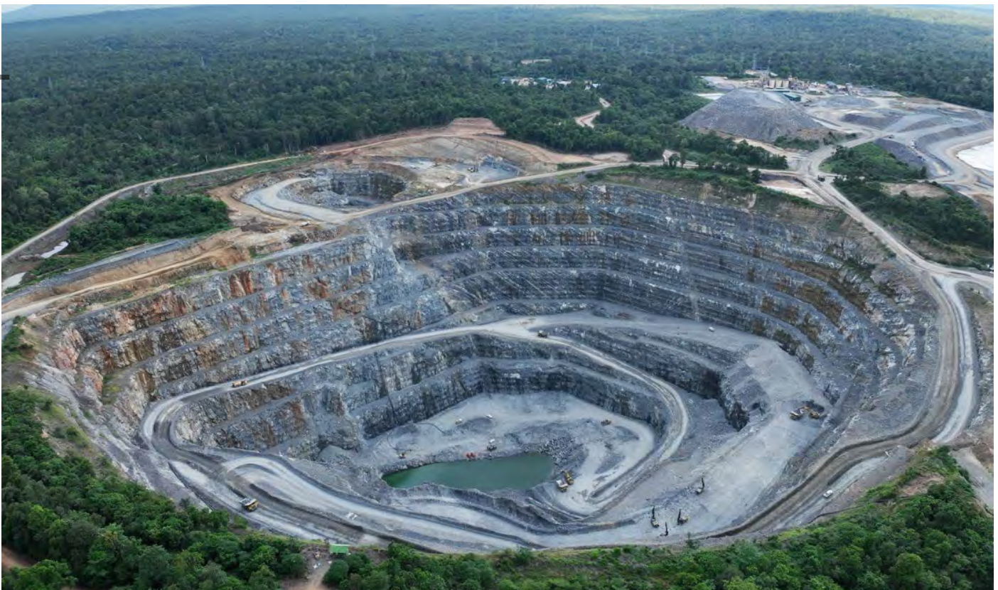
Figure 4 | Okvau Open Pit at July 2025
