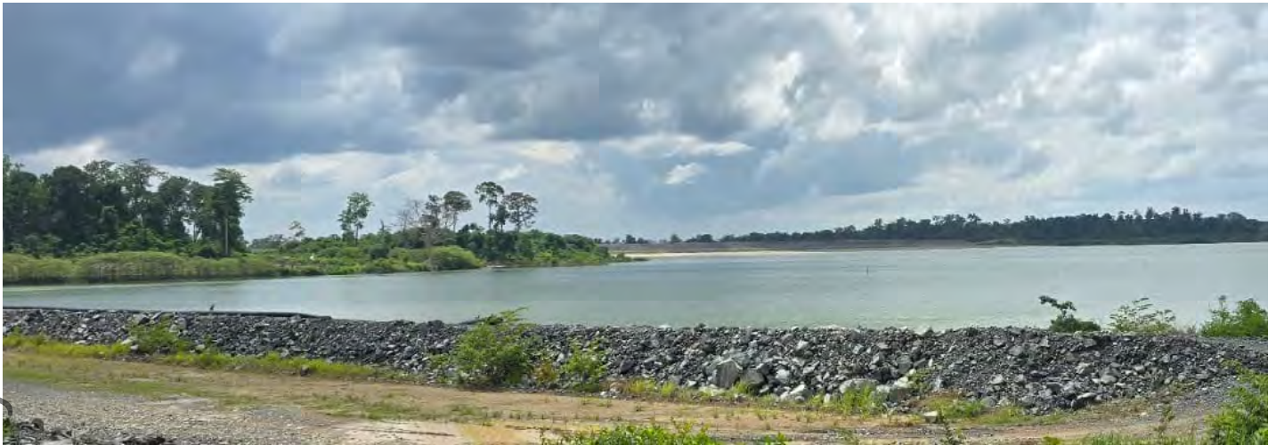
Figure 38 | Tailings Storage Facility at Okvau
