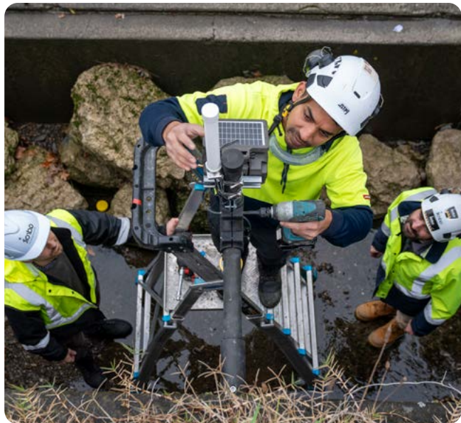
Technicians installing solar-powered sensors in Havelock North.
