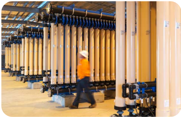
The Talinga Water Treatment Facility uses reverse osmosis to prepare water for beneficial uses such as crop irrigation.
