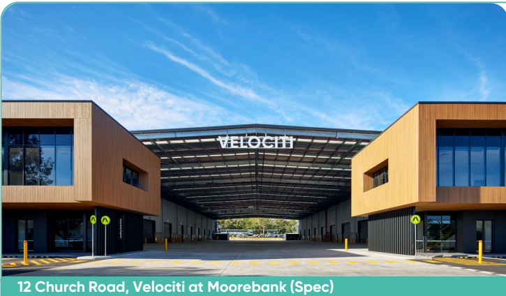
12 Church Road, Velociti at Moorebank (Spec)
